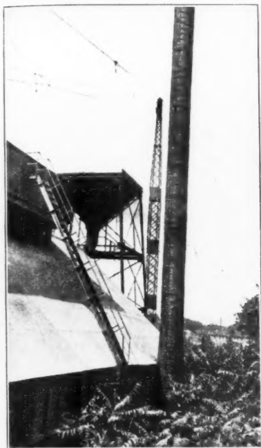
Steel Mast for Cableway
